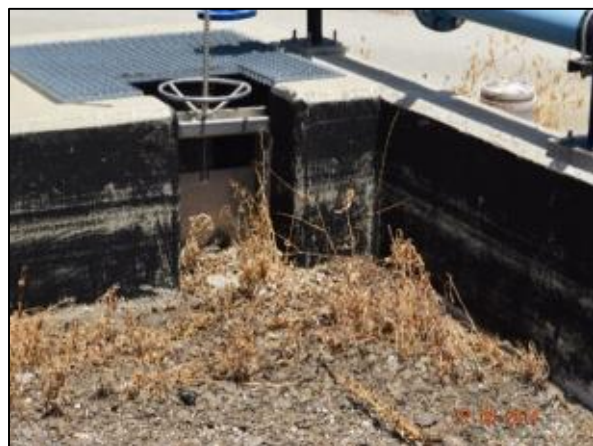
Figure 3-10 Supernatant evacuation system of the sludge: sluice gates
