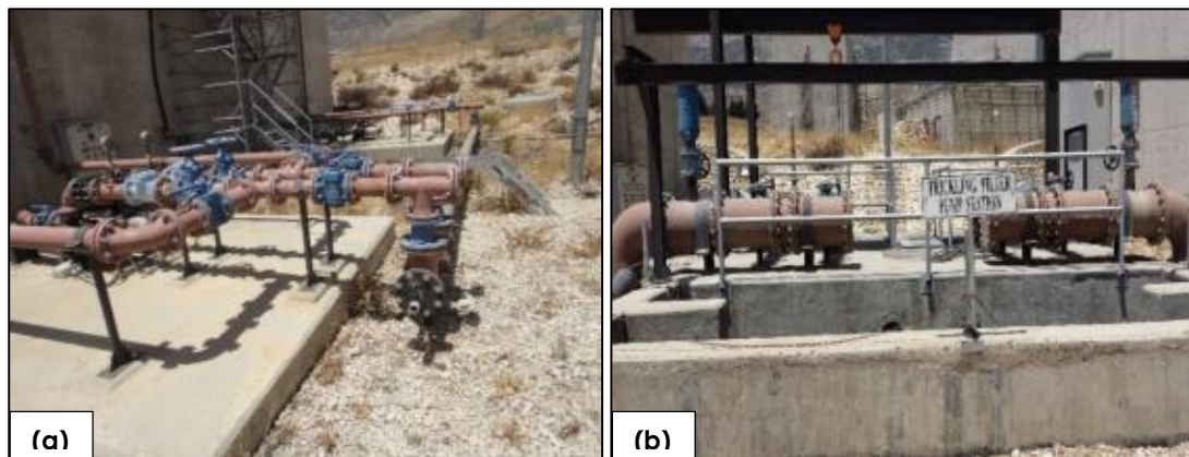
Figure 3-1 Pump stations for digester tanks (a) and Trickling Filter Unit (b)
