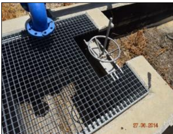
Figure 3-10 Supernatant evacuation system of the sludge: sluice gates
