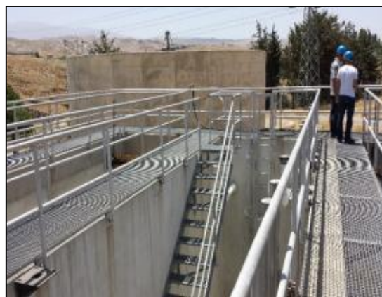
Figure 3-12 Safe Catwalk and Ladders
