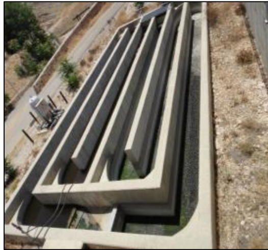
Figure 3-8 Chlorine Contact Tank
