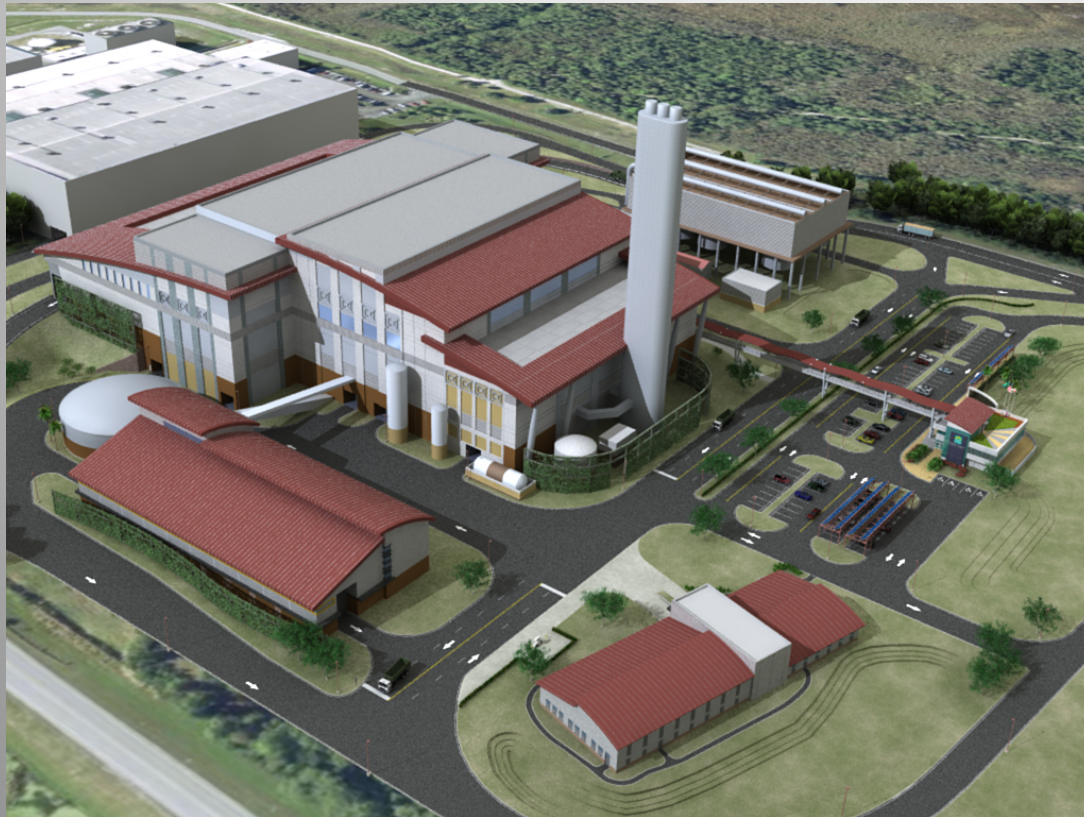
Three Unit, 3,000tpd Mass Burn 100MW Facility
