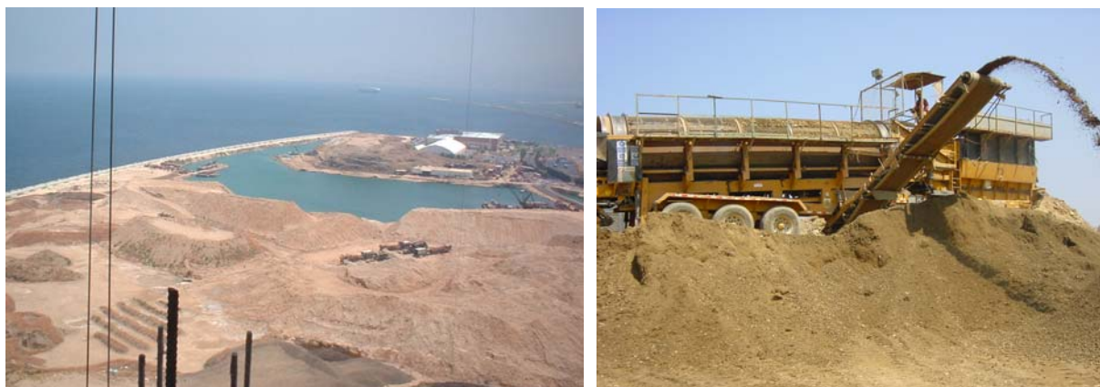
Photo 1 Rehabilitation Works at the Normandy Dumpsite in Beirut
